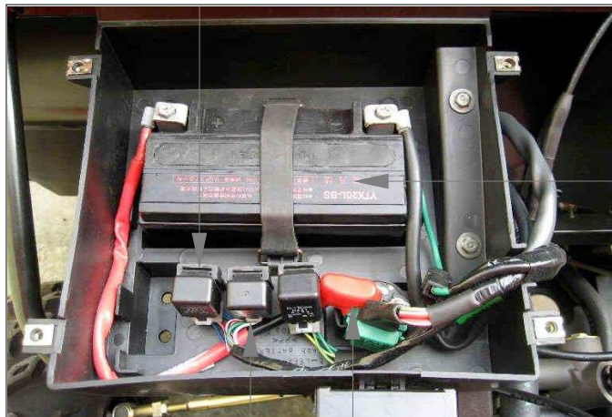
Hi Beam Relay
